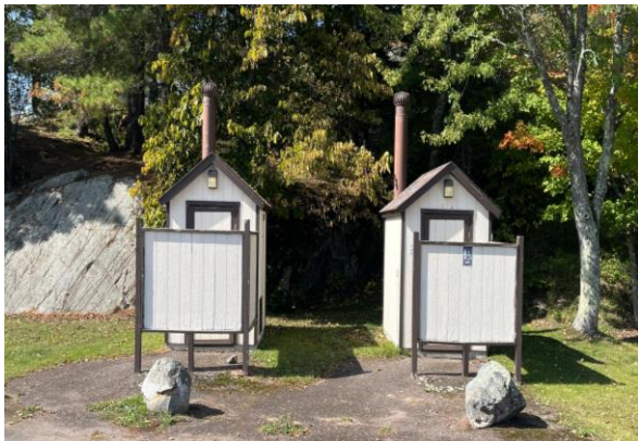
Lake Gogebic Vault Restrooms Prior to Replacement
