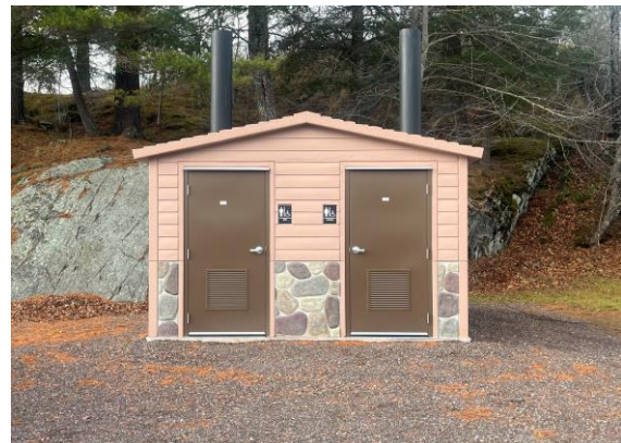
Lake Gogebic Vault Restrooms After Replacement
